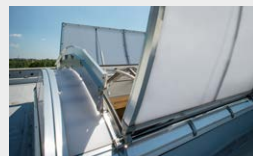
SMOKE AND HEAT EXHAUST
