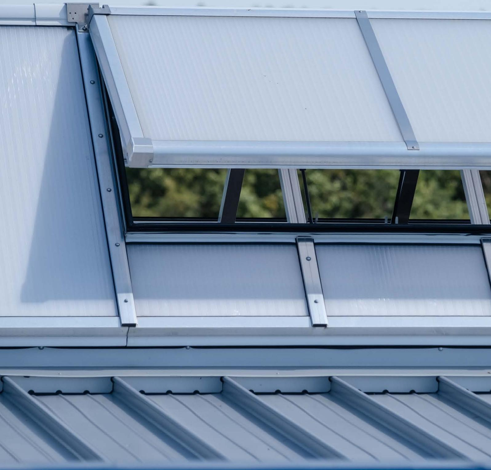
All smoke lift systems can be integrated as a single flap or as opposing double flaps. Similarly, it is possible to combine two flaps by arranging them directly next to each other. This flap combination acts as a natural smoke and heat exhaust ventilation device with a higher aerodynamic smoke extraction area, which is referred to as a tandem-serial single or double flap.
